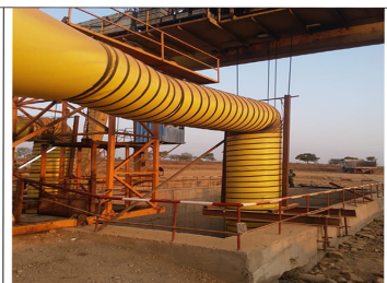
SEMI-RIGID PVC DUCTING
